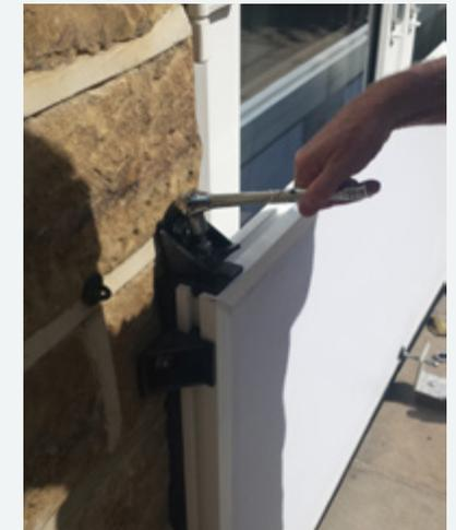
**Figure 10** Fitting new (taller but light-weight) barriers
